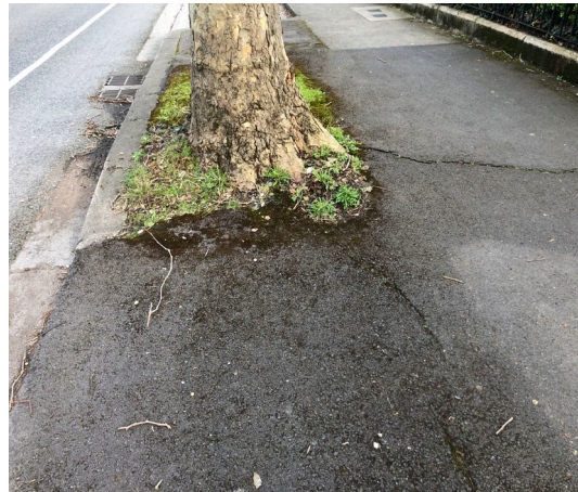
Image 10. Tree #603. Note bulging to tarmac from surface roots.
