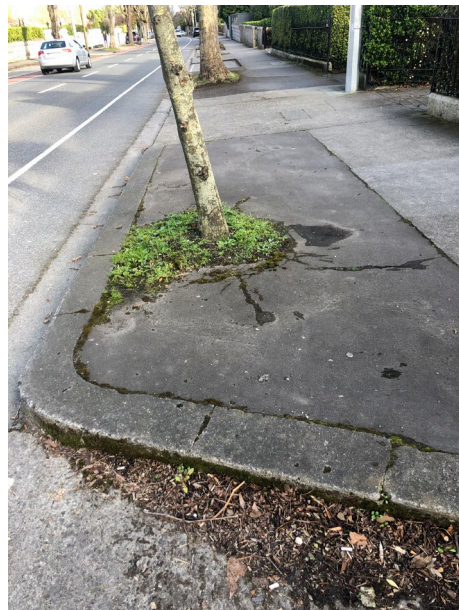
Image 8. Tree #604. Note bulging to tarmac surface.
