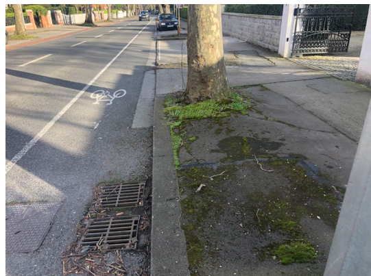
Image 3. Base of tree #607. Note bulging to tarmac from surface roots.
