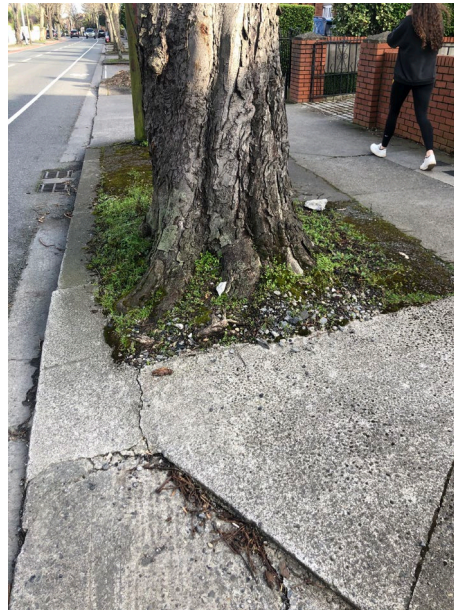
Image 6. Tree #605. Note bulging to paving and kerb
